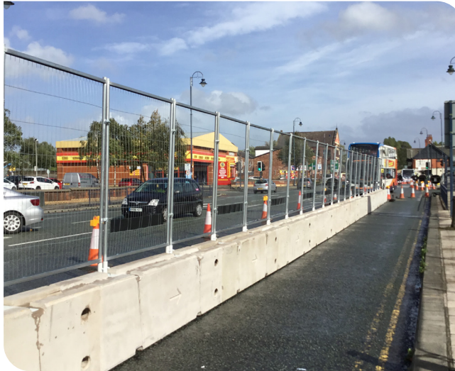
TVCB's with fence securing highway
